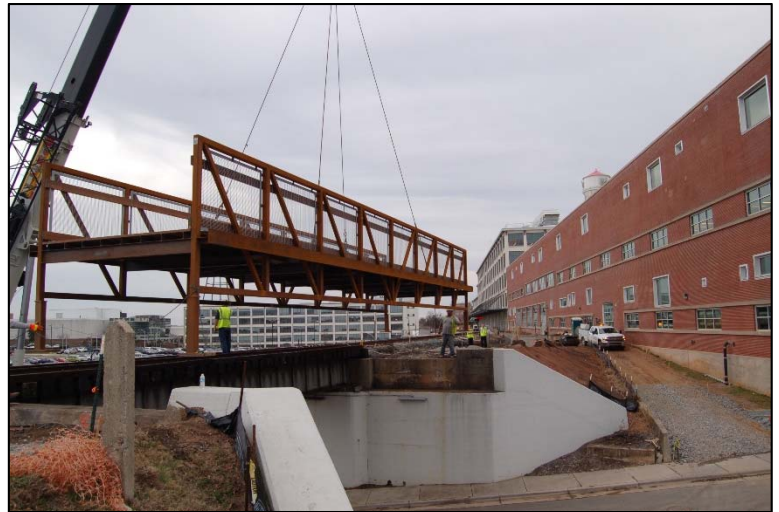
Figure 2: Long Branch Trail bridge installation over 7 th Street.
