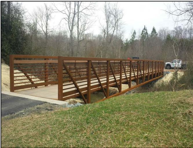
Figure 1: Cedar Trail Connector bridge over Muddy Creek.
